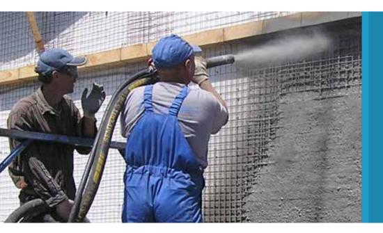
Dry mix shotcrete (gunite) is a versatile, flexible and economical method of construction and reconstruction. Properly chosen equipment allows to achieve good results in sprayed concrete application. TORNADO offers equipment, effective for the following types of work:
