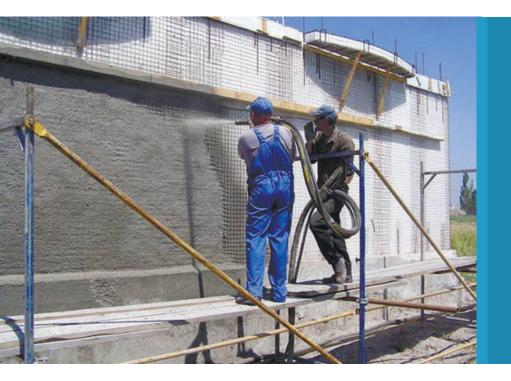
Wet mix shotcrete is a versatile, flexible and economical method of construction and reconstruction. Properly chosen equipment allows to achieve good results in sprayed concrete application. TORNADO offers equipment, effective for the following types of work:
